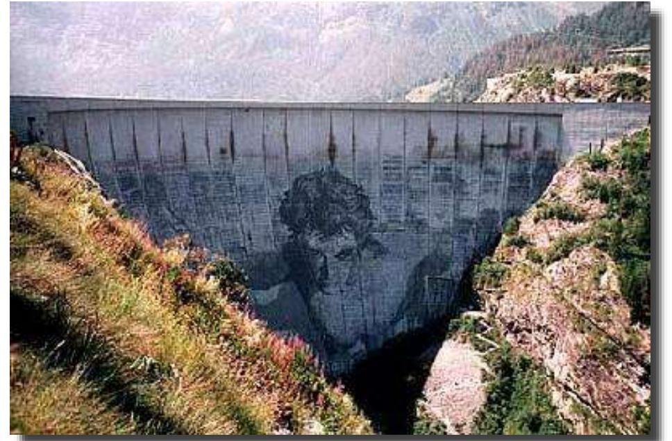
Tignes Dam, France, 180 m
