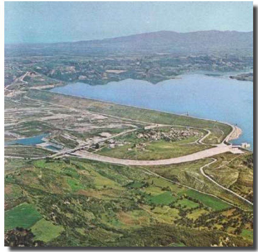
Pinios Dam, Greece, 50 m
