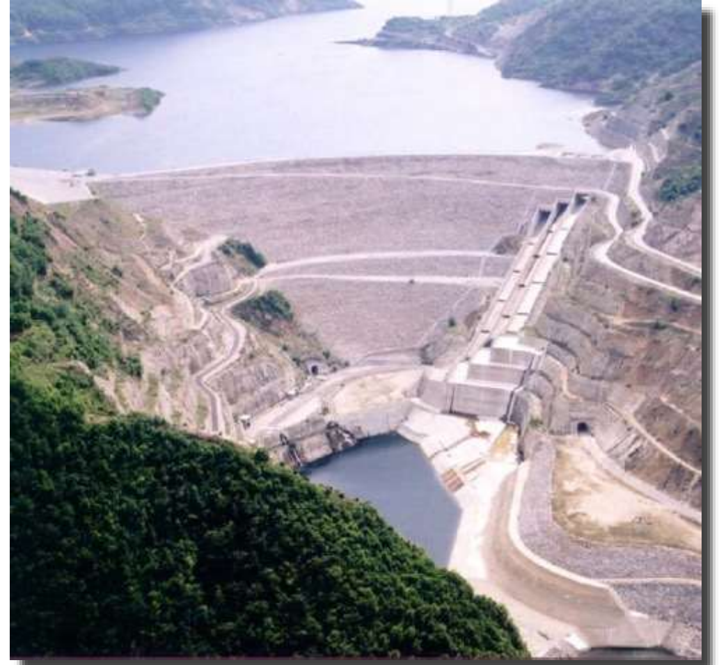
Thissavros Dam, Greece, 172 m
